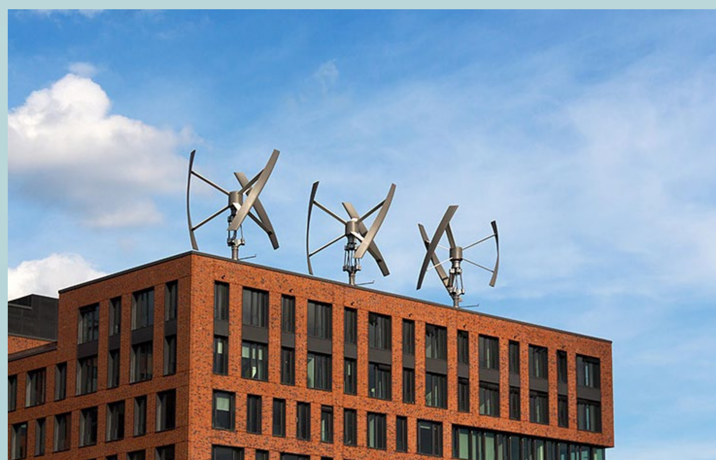
Fig 2: Darrius wind turbine mounted on building. [1]
